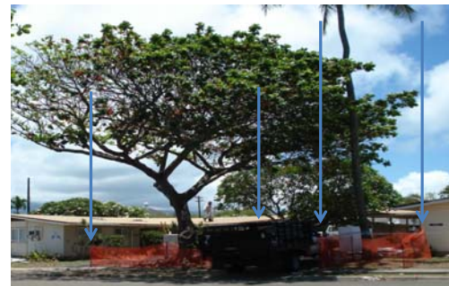
all non-paved surfaces under the trees are protected with construction fencing
